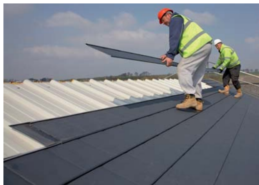
Below and right: Carrwood Park, Leeds. Meta-SlatePlus roofing system with barrel rooflights to a new building during and after installation with view from inside showing underside of AS35 panel.
