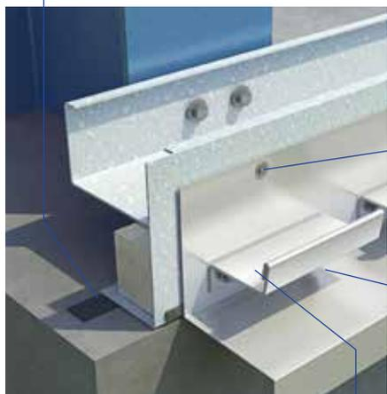
3. Align and fix the drip flashing using low profile fasteners. Form 100 mm lap joints and seal with two runs of butyl sealant.
