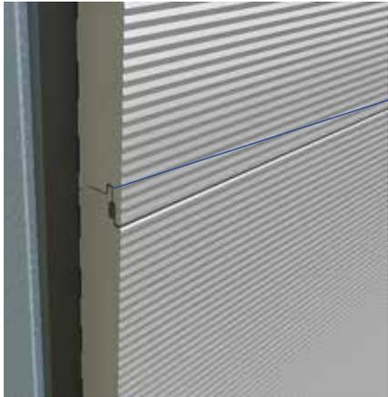
11. Bed proprietary joint filler piece in gun-grade sealant at end of panels at the vertical joints.
